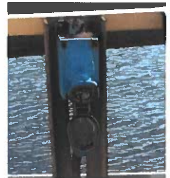
Above: A broken marine electrical plug, and electrical runs not maintained in accordance with NFPA 70.
