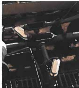
Above: A broken marine electrical plug, and electrical runs not maintained in accordance with NFPA 70.
